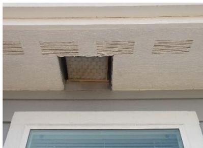
Outside Air Vent on the underside of the overhang (Cover is off to show the air filter inside)
