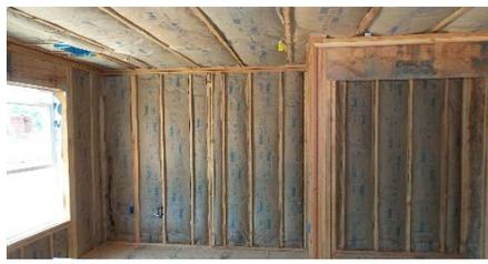
Ceiling and Exterior Wall Insulation
